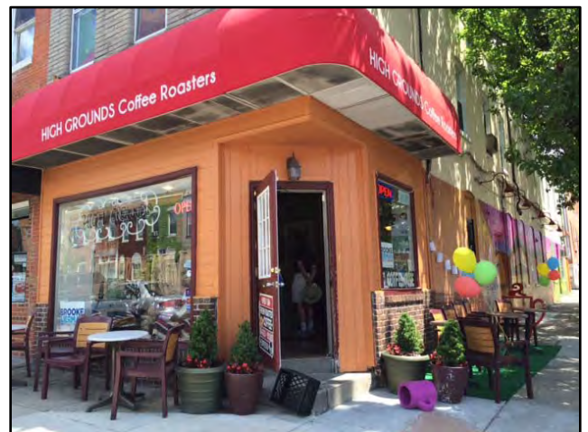
Completed awning at High Grounds Coffee Roasters, 3201 Eastern Ave.
