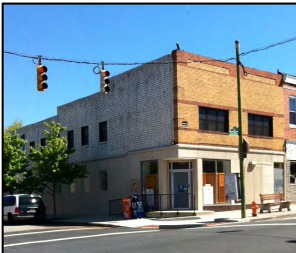
Before image of 3200 Eastern Avenue.
